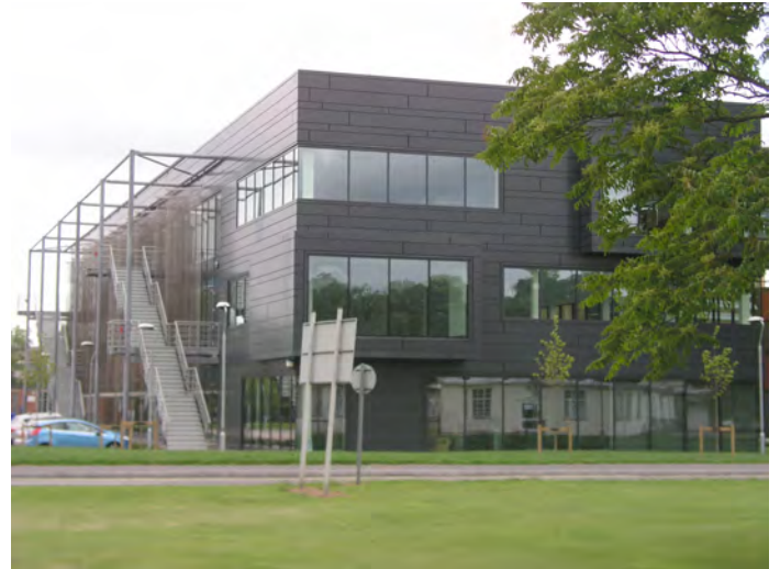
Reading Enterprise Centre with wire mesh solar shading
